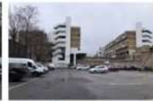
02. Thomas Lane car park (west view)
